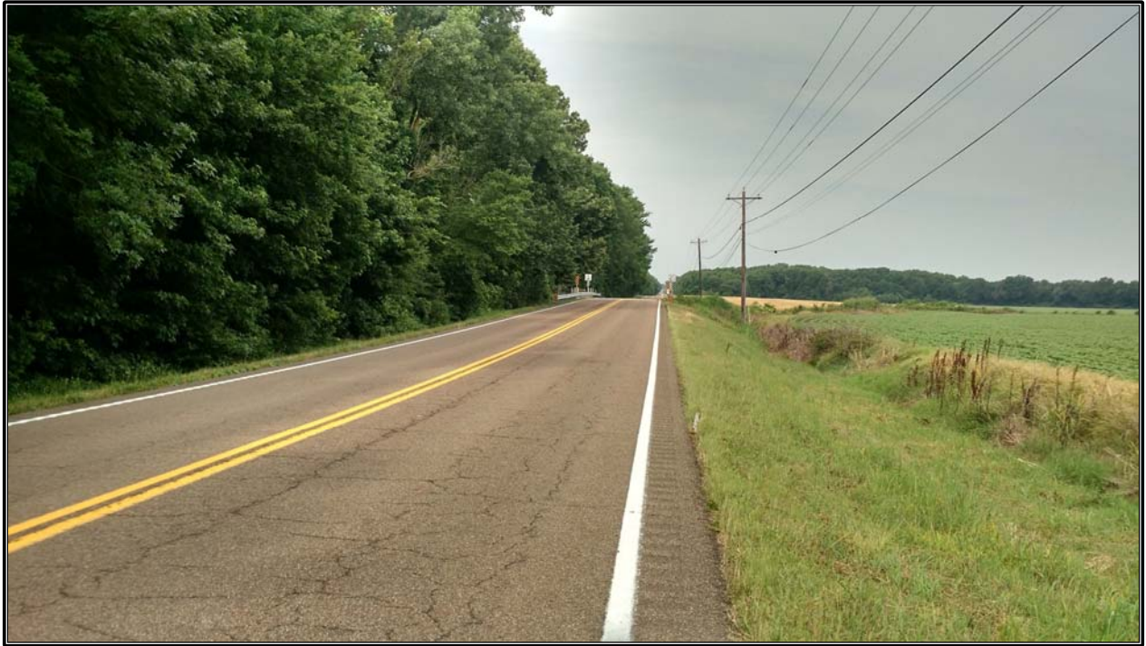
Figure 2. SR 1 within the APE. View is looking west from the eastern edge of the APE.
