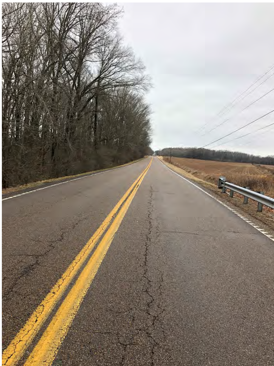
Looking West from Bridge
