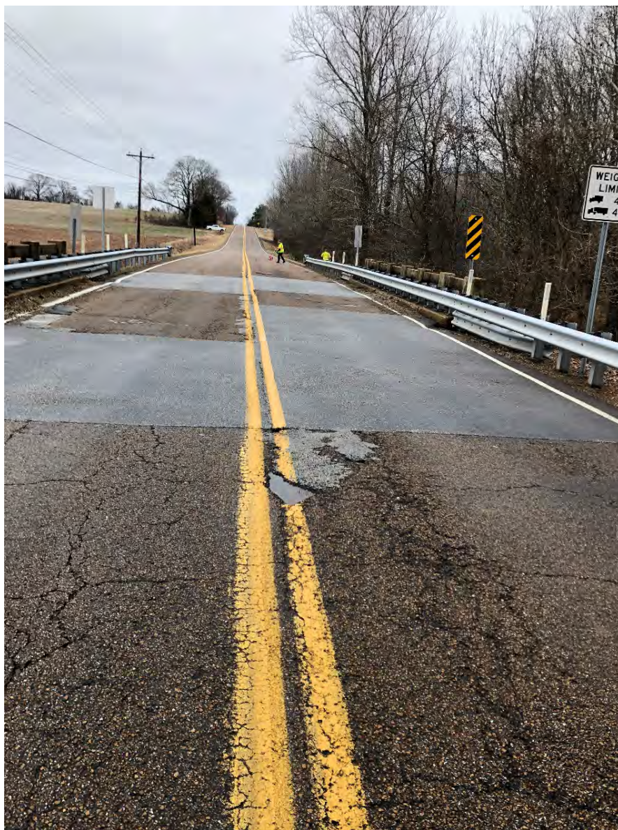
Eastbound Approach to Bridge
