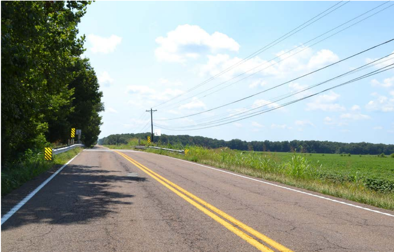
Figure 4: View southwest toward the bridge.
