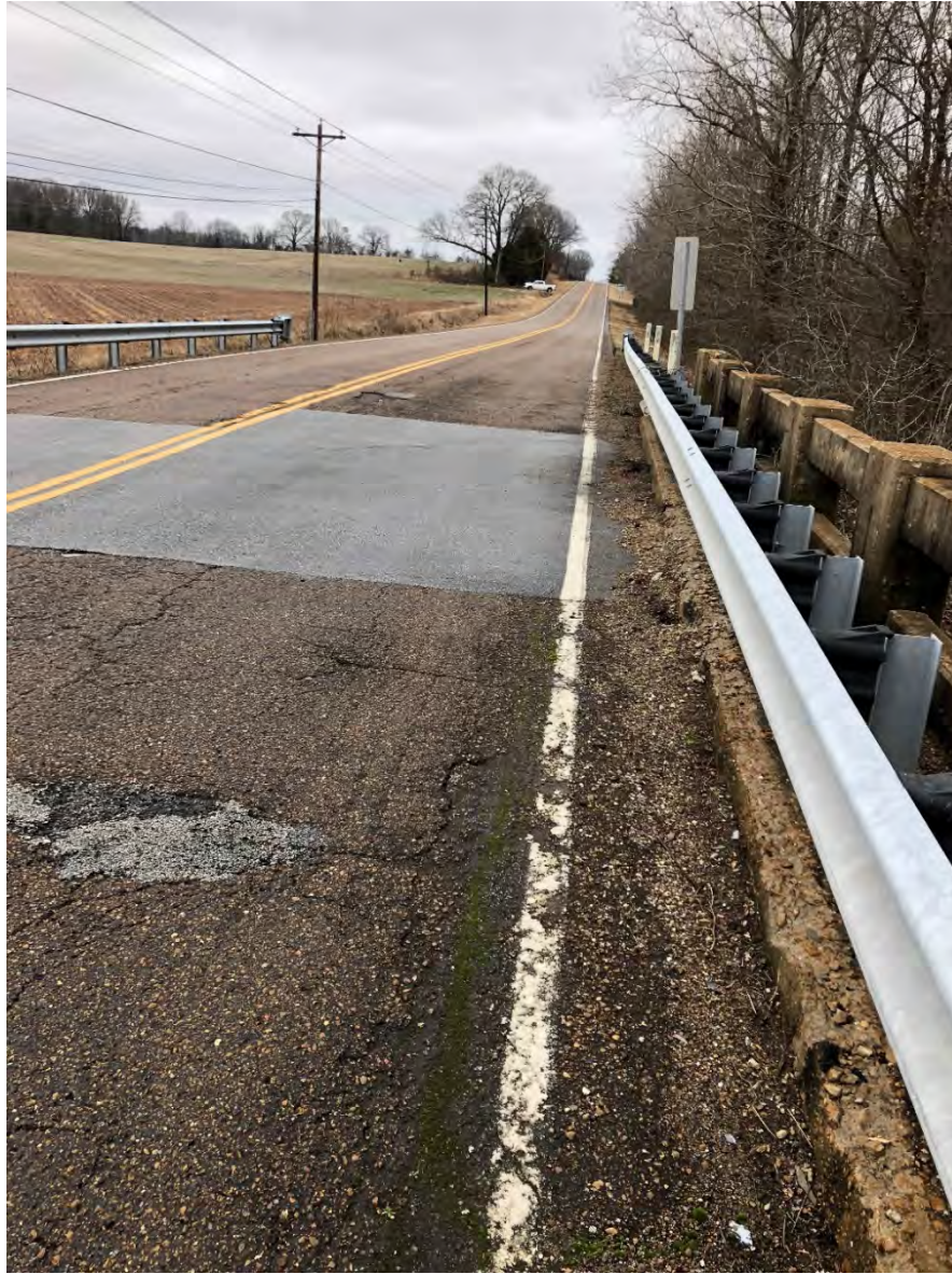
Looking East from Bridge
