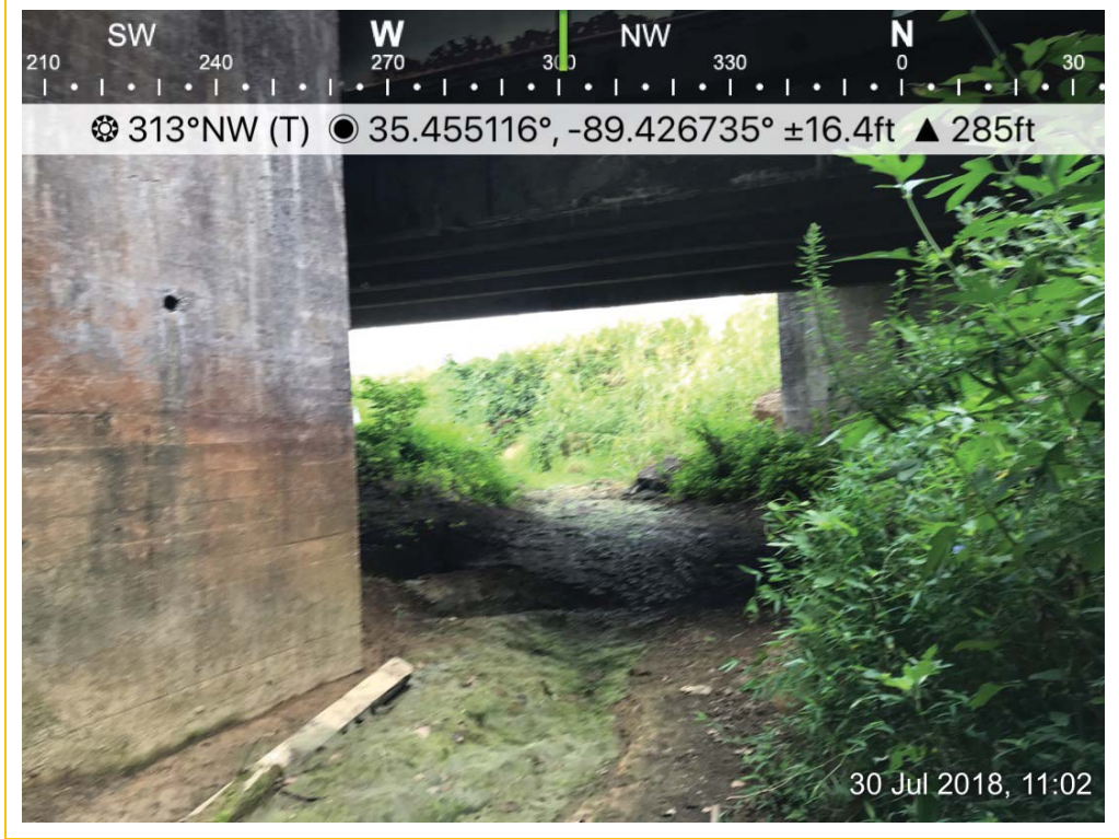
Photo 2. STR-1 – Looking downstream
