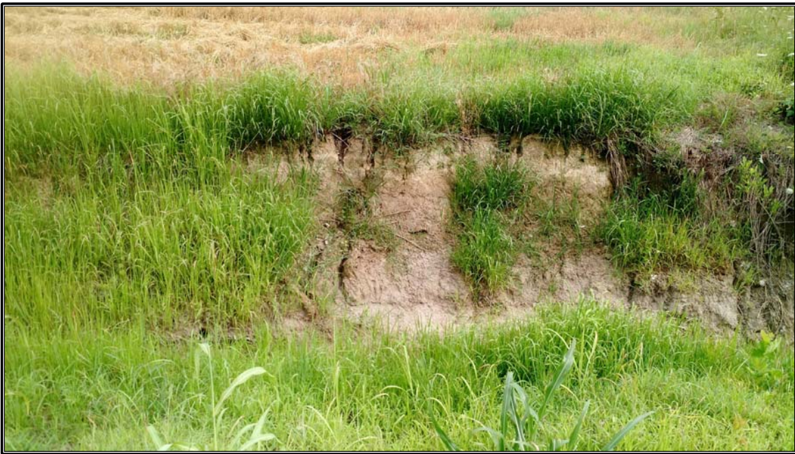
Figure 12. Exposed cut bank in the northwestern quarter of the APE.
